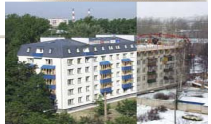
Fig.10.0. A model of refurbished joint dwelling Source: Pedro Guertler and Winton Smith, 2006 Association for the Conservation of Energy report
